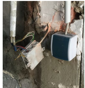
Abb. 6 Defekte Installation
